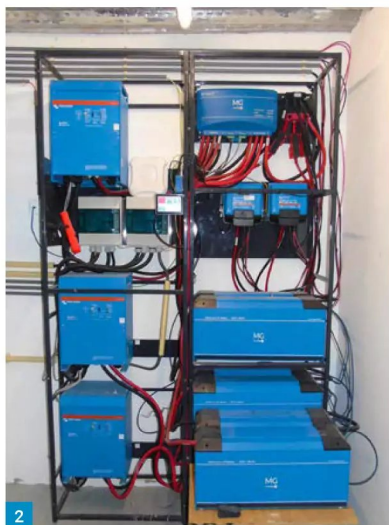
Fig. 1: The PJ4MM station is located well away from neighbours on a hilltop in the centre of Bonaire. Fig. 2: The battery room at the PJ4MM station. Fig. 3: Martin Moens PJ4MM in his VHF/UHF shack. Fig. 4: The InnovAntennas 8-element 70MHz LFA Yagi, beaming at Europe. Fig. 5: Top to bottom: 23cm 23-ele, 70cm 38-ele, 2m 9-ele and 6m 7-ele Yagis. Fig. 6: Martin building the 6m H-frame. In the background the 24m heavy-duty tower.
